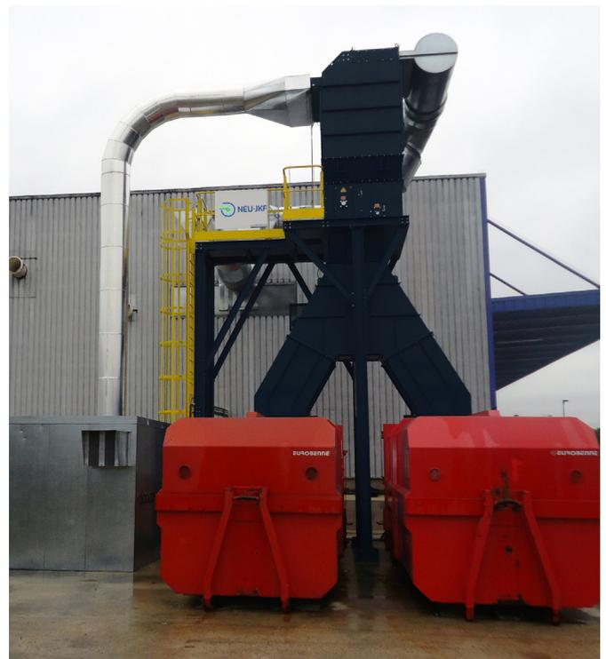
Pneumatic waste collection system in cardboard company with SEPAROJET M and CHOPPERLINE
