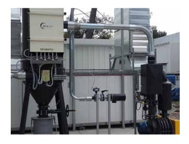
A centralised extraction system effectively sucks up the dust generated throughout your process, providing complete cleaning of the floor, equipment and production machinery.
