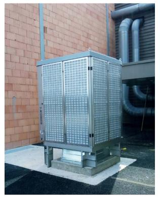
40,000m<sup>3</sup>/h of air is reintroduced, partly through the gutters and partly through textile ducts. This operation, the dynamic compensation via channels, guarantees working comfort for the operators. The originality of the solution lies in the fact that the air compensation system is equipped with an air cooling system that can be activated in case of very high temperatures. The system thus protects the operators while guaranteeing them working comfort.
