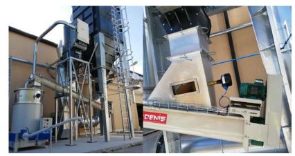
The system is controlled automatically. The machine suction ducts are equipped with an electro-pneumatic flap. The opening and closing of each door is controlled by the machine start-up.
