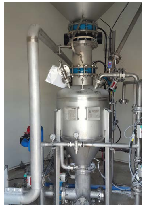
NEUPHASE conveying by blow tank.
