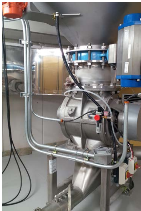
Dilute phase transfer, suck blow system for powder
